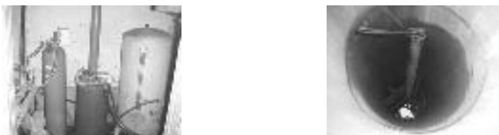
*Figure 3.1: Typical picture of a hydrofore (left) used to pump water from a well (right), taken during the sampling campaign.*
