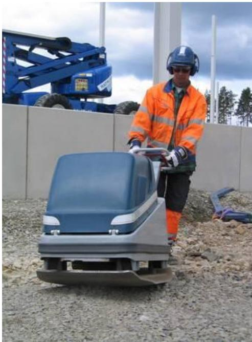
*Figure 10. An example of a soil compactor and how it is used (Swepac International AB 2008).*
