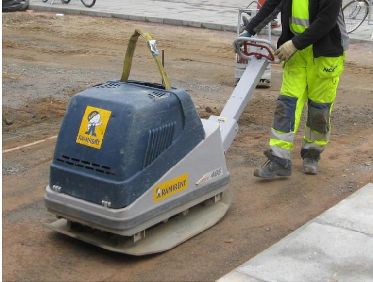
*Figure 12. The FB-455 soil compactor in use with the transport textile strap erected.*
