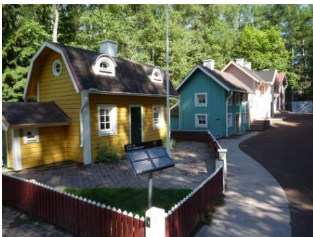
Figure 2: Troublemaker Street. Houses on the outskirts of a forest, with fences and signs. Visual documentation 2010.
