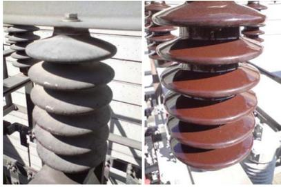
Fig. 3. Insulators before (left) and after (right) cleaning with the QM.
