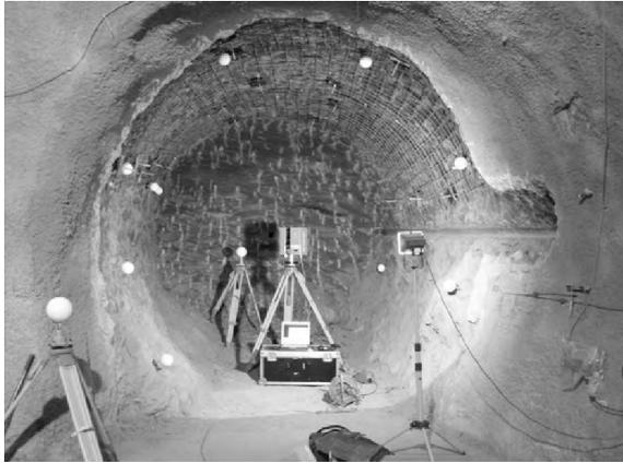
Fig. 3 Laser scanning of excavation surface of tunnel
